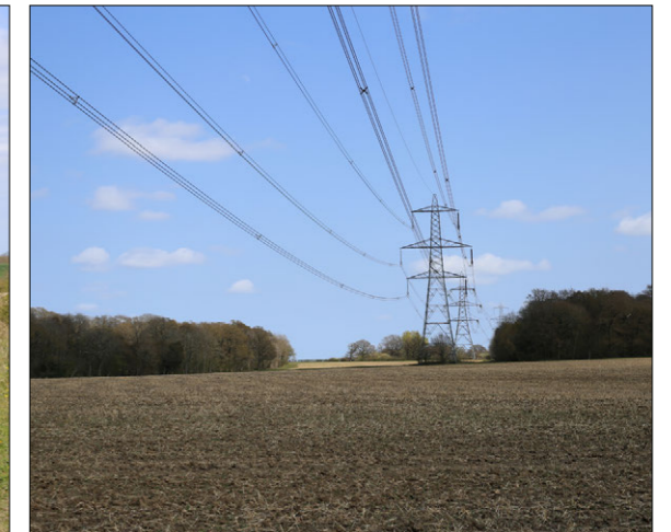
View east from pylon approximately 100m south of the viewpoint
